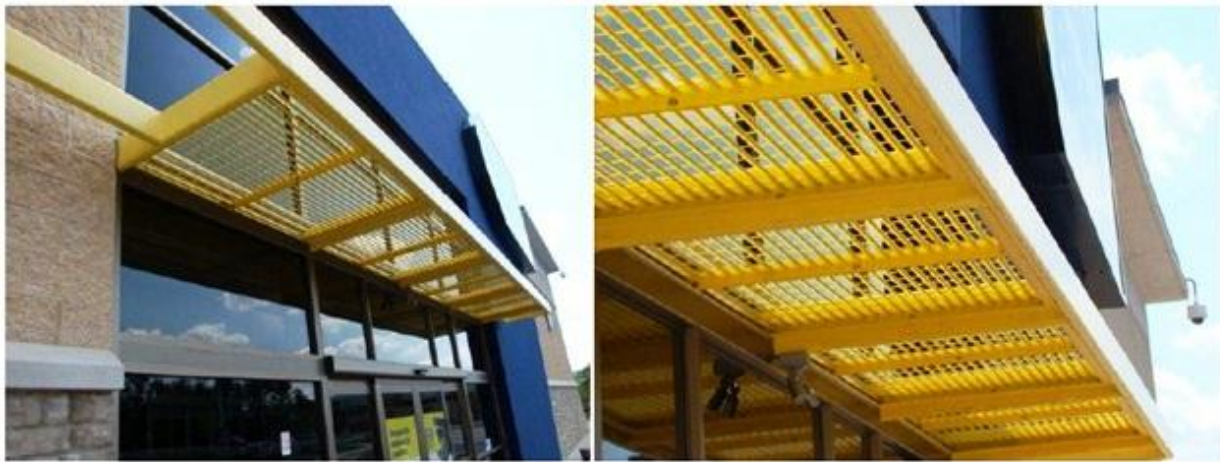
Fig 8 : Samples of the solar shades that could be used to minimize the direct solar irradiance
